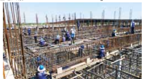
● 鋼筋作業 Reinforced work
