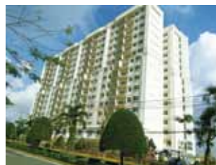
● 海悅住宅大樓 Hai Yatt Residential Building
