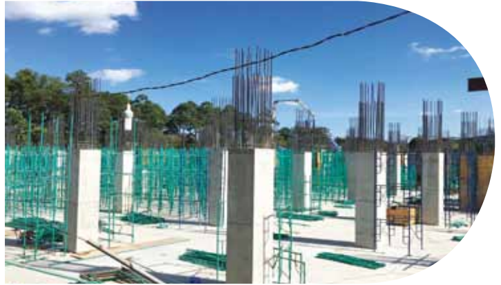
● 鷹架作業 Scaffolding
